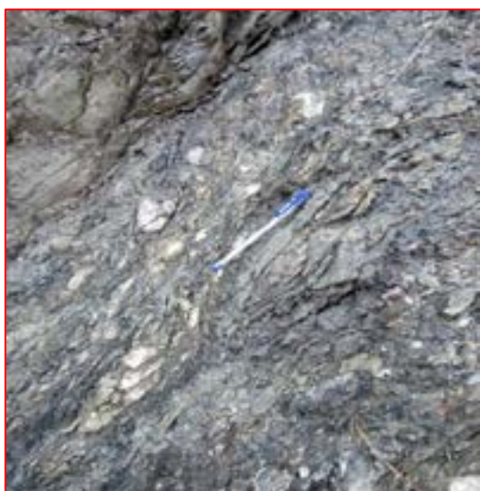
Fig. 8. Crushed phyllite/schist in MBT at Shahanshahi Ashram, now concealed under a retaining wall.
