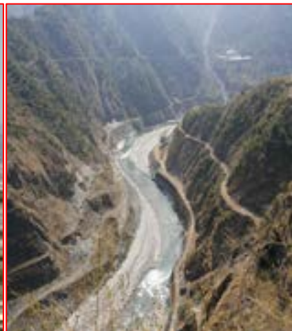
Fig. 7. Lakhwar dams site on 800 m thick dolerite sill in Yamuna valley.
