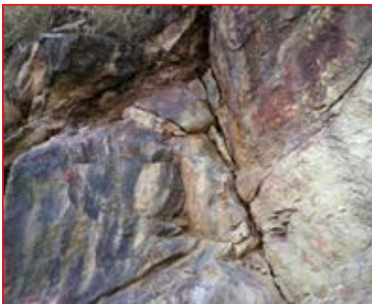
Fig. 12. Polished faulted surface, slickensides, in quartzite near gossan.
