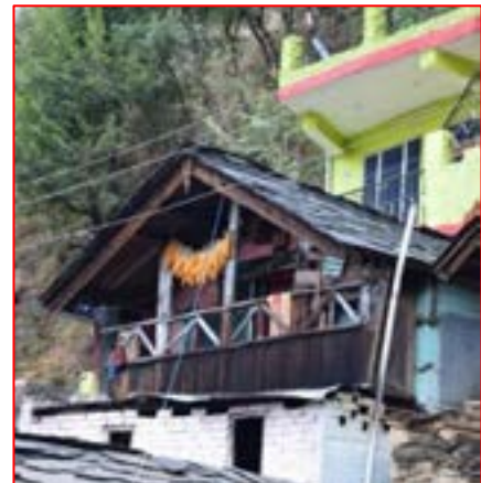
Fig. 14. A modern cement house above a traditional house.
