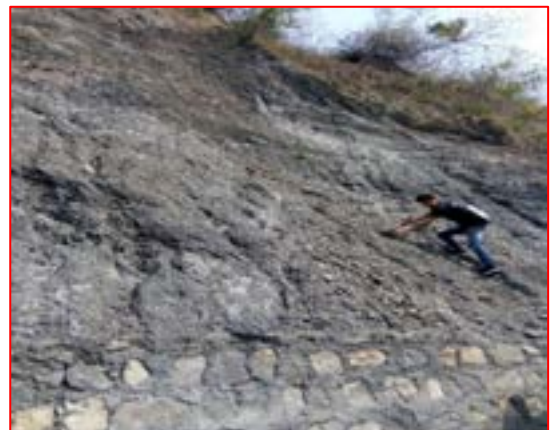
Fig. 13. Burnt zone in Lesser Himalaya in MBT zone in Shahanshahi Ashram, Rajpur Road, Dehradun.
