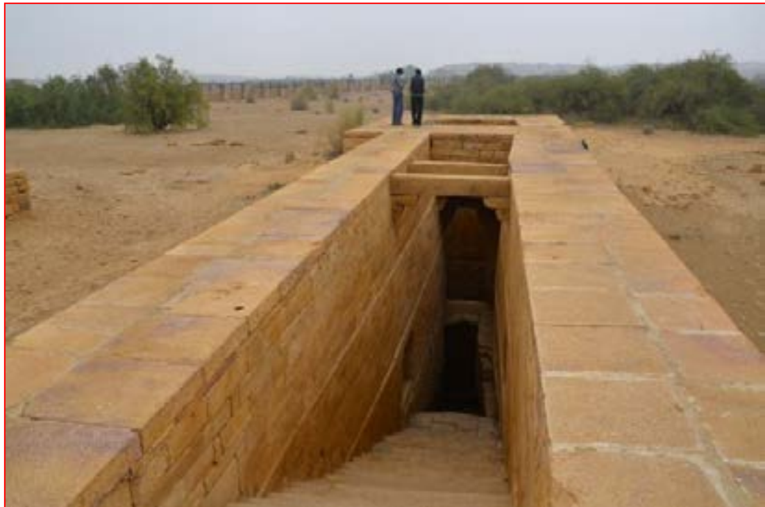
Fig. 16. Traditional rainwater harvesting structure - A step well [recently renovated] leading to the deep-water table in the middle of the desert environment at Kuldhara, Jaisalmer Basin, Thar Desert.
