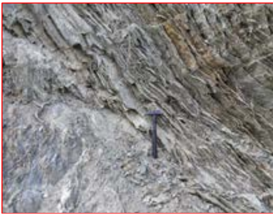
Fig. 11. Gossan in brittle fault zone near Yamuna Bridge.
