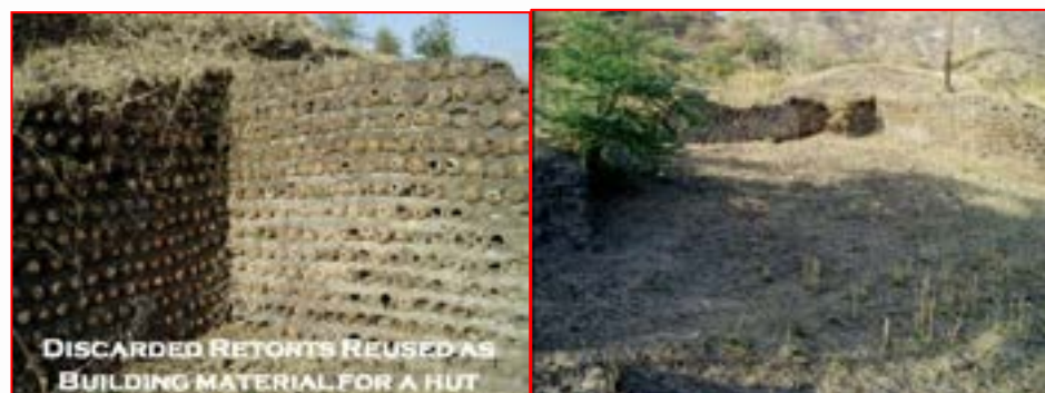
Fig. 4: Discarded clay retorts used for smelting were reused as a construction material for the huts in this area. Kumar (2017).
